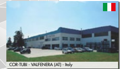
COR-TUBI - VALFENERA (AT) - Italy
